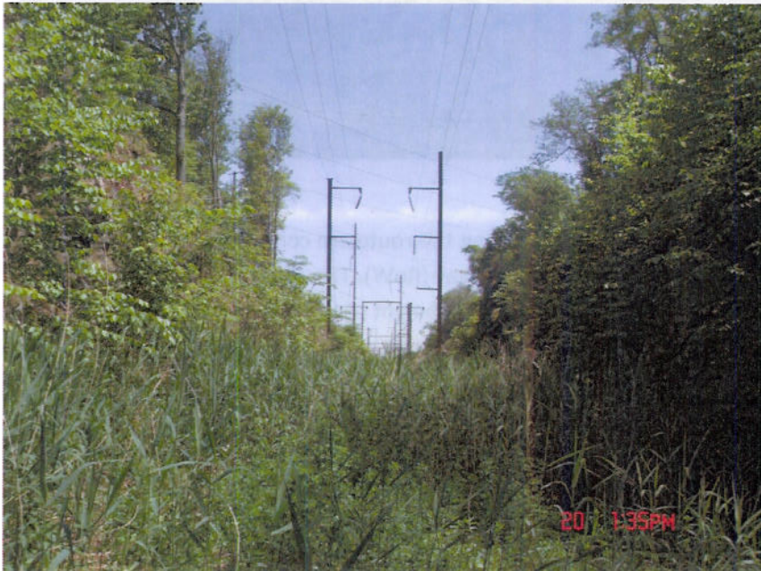
Figure 1 - Existing Transmission Right of Way
