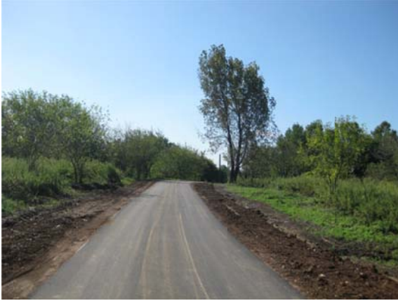
Section of Delaware River Trail
