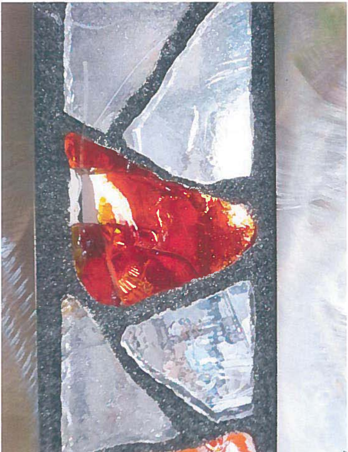
Broken glass unit
