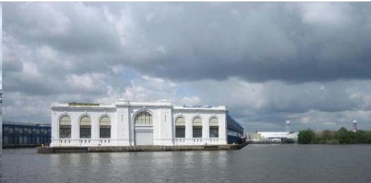
Port Slips – Pier 78
