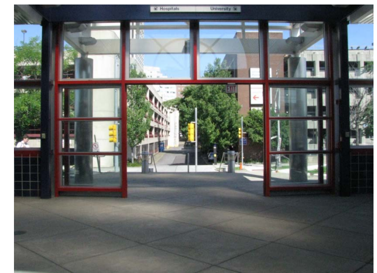
HEAD HOUSE - MAIN ENTRANCE (WEST WALL)
