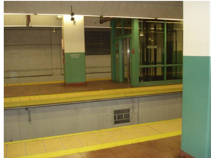
PLATFORM ELEVATOR VIEW
