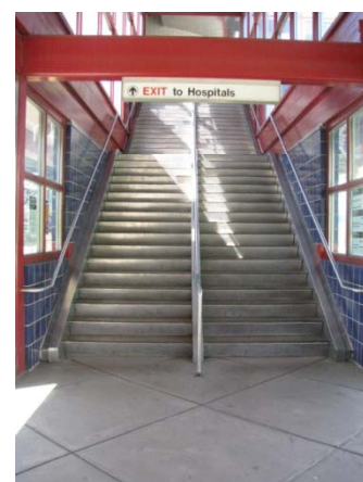
STAIR 1 VIEW AT PLATFORM
