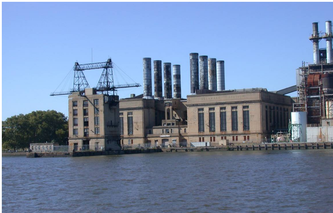
Delaware Generating Station—One of many (former) industrial sites that should be evaluated as reuse/redevelopment candidates.
