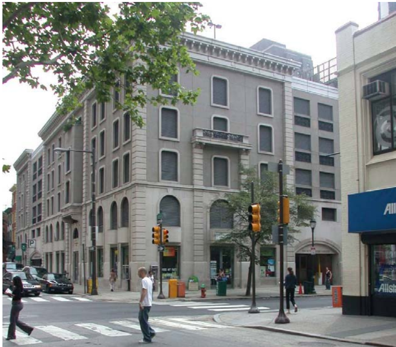
This well-designed parking garage in Rittenhouse Square minimizes adverse impacts on pedestrian safety and comfort.
