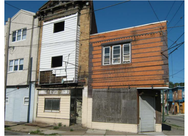
Vacant buildings at SW corner Point Breeze Ave. & Morris St.
