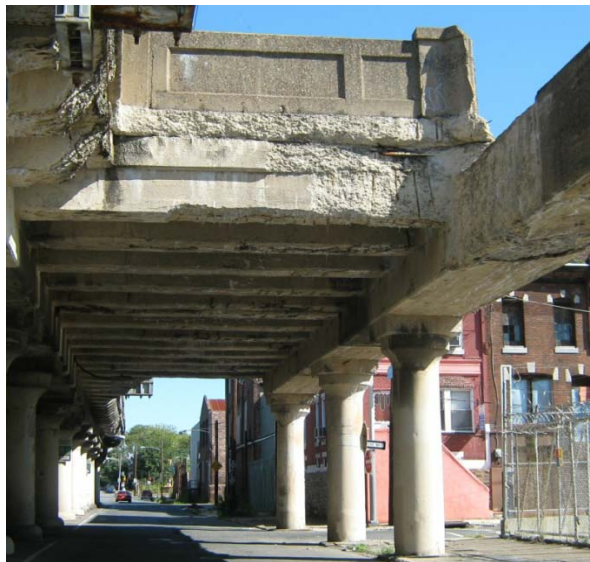
Damaged sections of railroad structure on 25 th St. near Federal St.
