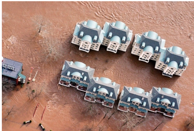
NEW HOPE, PA CONDOMINIUMS INUNDATED DURING THE JUNE 2006 FLOOD. THESE RESIDENCES WERE BUILT BETWEEN THE DELAWARE CANAL AND RIVER, IN A FRAGILE ENVIRONMENT SURROUNDED BY WATER WITH NO RIPARIAN BUFFERS OR PROTECTION FROM OR FOR THE RIVER.
