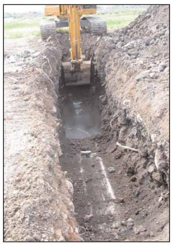
**Photograph 66:** Action shot of trackhoe excavating SRT-3 showing concrete floor, concrete footer, and demolition rubble associated with Sugar Refinery. View facing east (May 2008).
