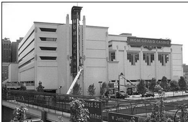
Detroit’s MGM Grand casino reinforces drive-up customers’ sense of security with its fortress-like appearance and direct access from the parking garage to the gaming floor.
