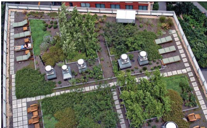
Green roofs help buildings achieve better energy efficiency by reducing heating and cooling needs, as well as aiding in stormwater management through increased vegetative surfaces. They also decrease heat island effect through absorption of solar radiation.
