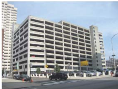
15th and Spring Street Parking Garage: 1,050 spaces
