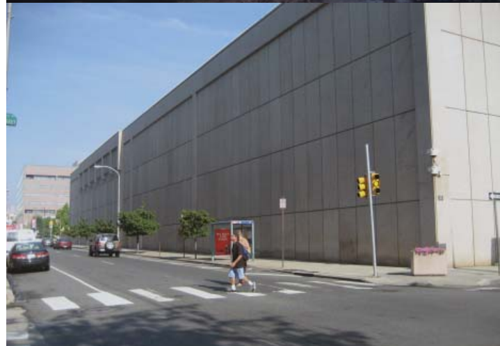
The United States Mint, 4th and Arch, serves as a local model of a mega-block structure. The large expanse of blank walls in the midst of an urban setting serves to detract from the pedestrian environment and creates a physical and psychological barrier between the neighborhoods north of Old City and Society Hill.
