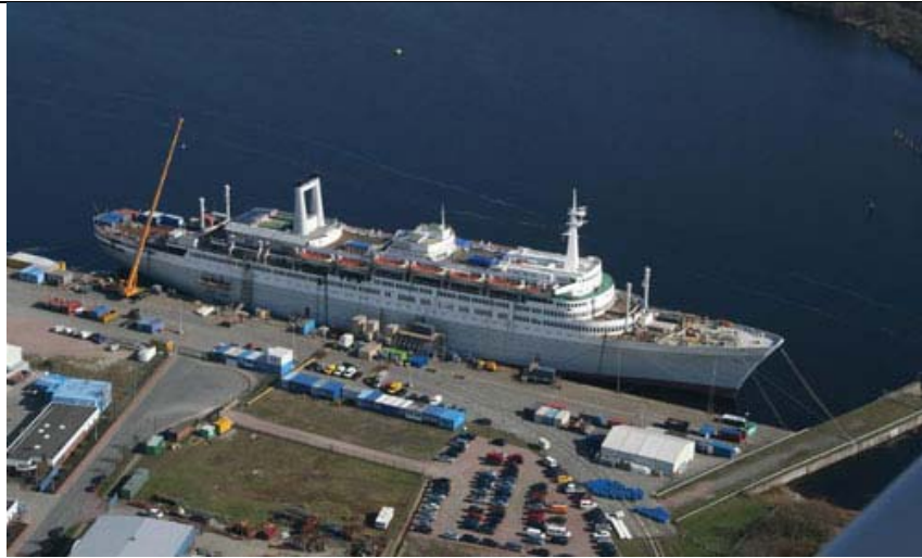
The Rotterdam undergoing restoration in Wilhelmshaven, Germany, 2007.
