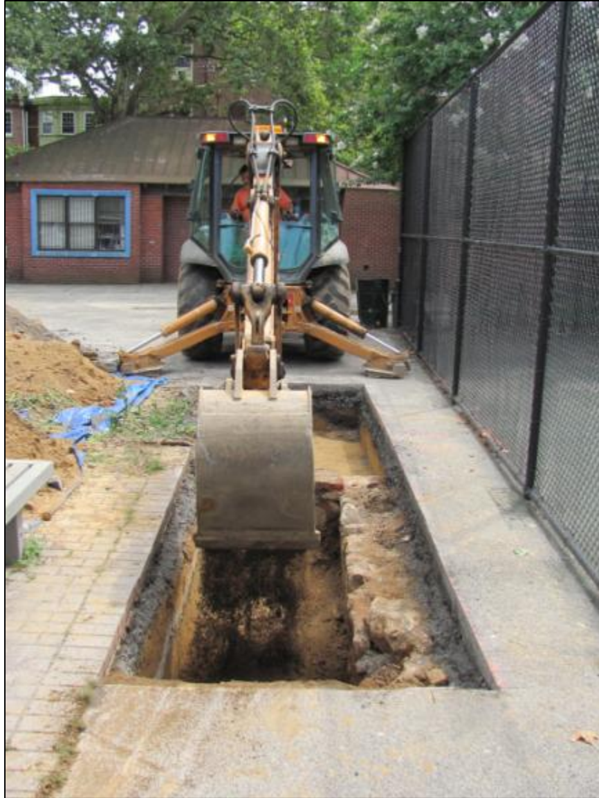
Figure 3.7 Backfilling a trench after excavation was complete.
