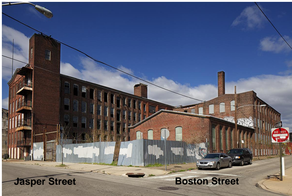
East-to-west view of 1817-41 York Street
