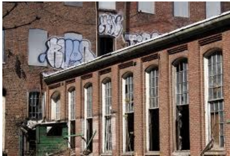
First-floor courtyard windows, April 7, 2012
