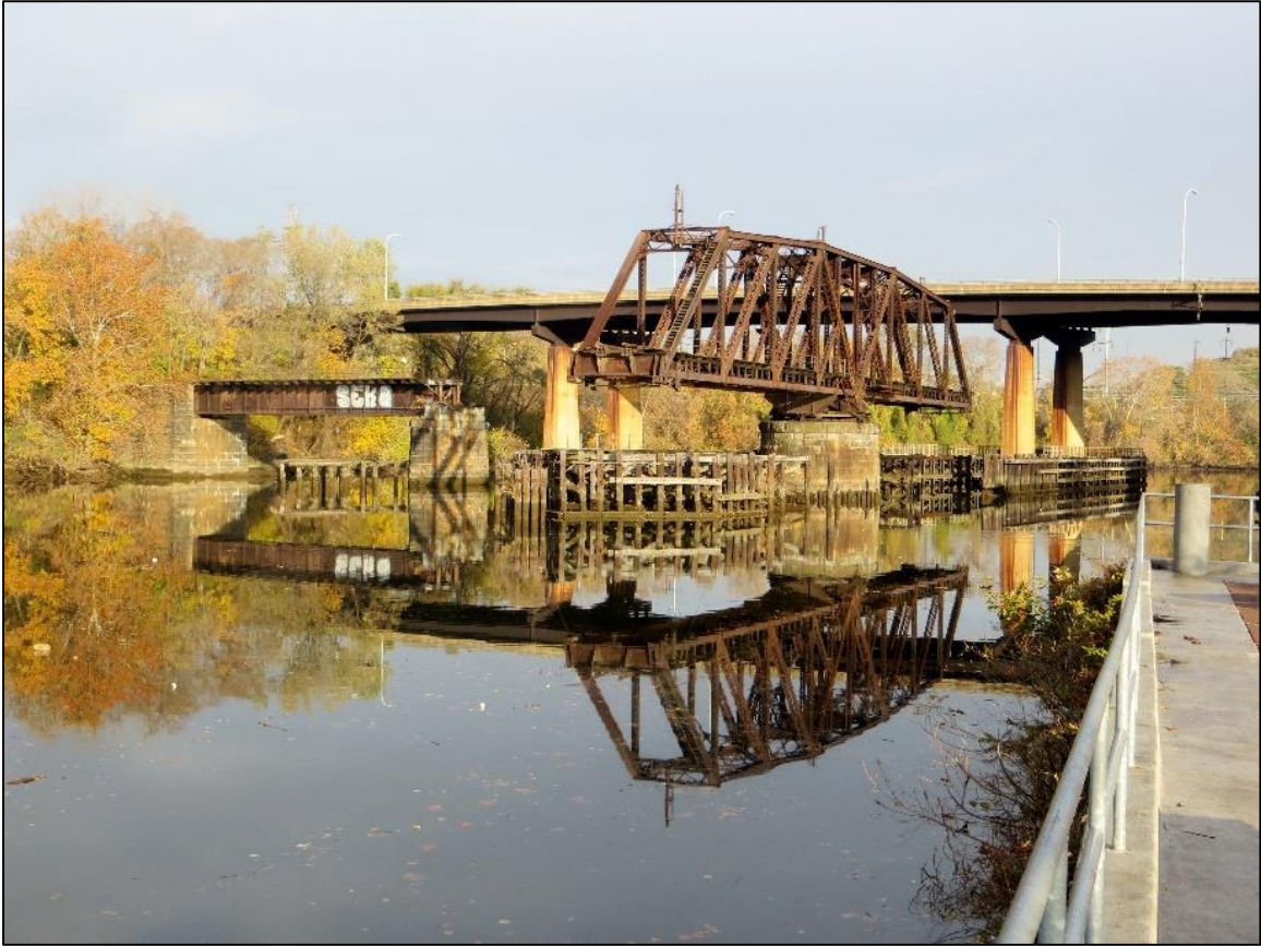
Exhibit 11 Over the River - Existing Conditions
