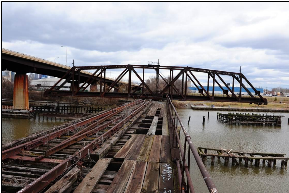
Exhibit 3 Current Conditions - Schuylkill River Rail Bridge
